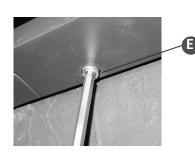
**Step 5** – Mount the luminaire on the bracket and secure Eseta with two screws **E** on the bottom of Eseta to complete the installation.
