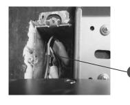
Step 4 – Connect wiring to customer supplied junction box **D**. Connect the black wire to hot wire, connect the white wire to the neutral, connect the red wire¹ with ON/OFF switch wire, and connect the green wire to the ground.
