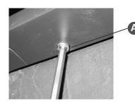
**Step 1** – Remove two screws **(A)** on the bottom of Eseta and remove mounting bracket on the back of the luminaire.
