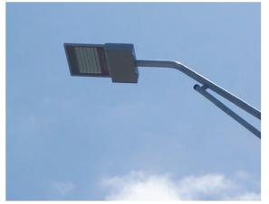
Leotek's LED street lights are a direct replacement for traditional HID cobra head style fixtures. They mount directly on to the existing mast arm.
