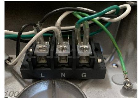
**Step 5** - Connect service lead wires to terminal block (black service lead wire to "L" Line, white service lead wire to "N" neutral, and green ground wire "G" to ground).
